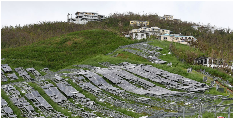
Solar farm on St. Thomas destroyed by a hurricane. (FEMA photo by Jocelyn Augustino)
