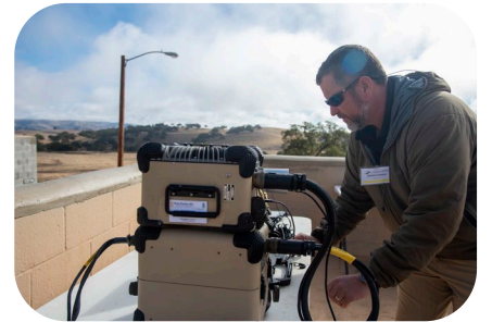
K-03: Bren-Tronics set up their austere battery packs for uninterrupted power.
