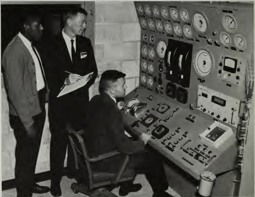
Control console for the turbojet test cell in the Jet Engine Laboratory
