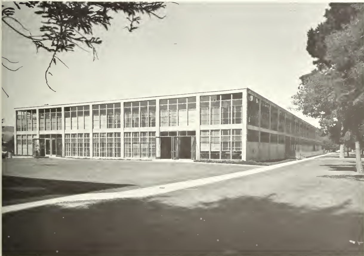
Electrical Engineering Laboratories
